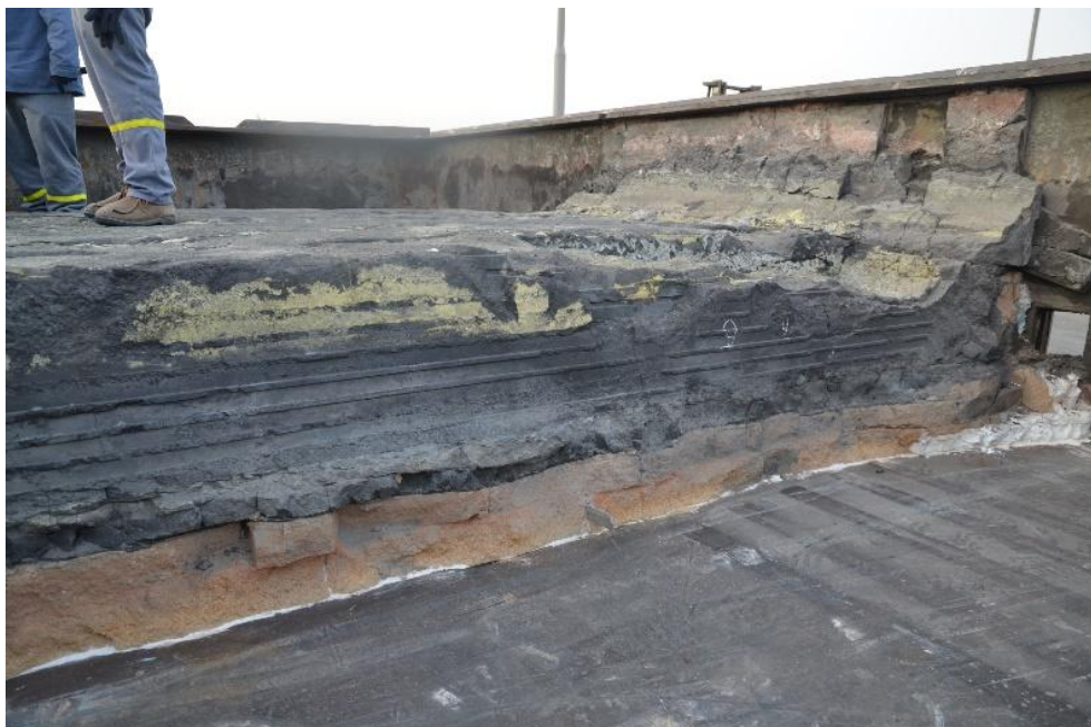
Figure 5. Sub-cathodic lining condition in the copper insert pot.
